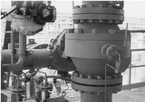
Coke particles suspended in gas travel through this 16" 300# VCM Furnace Isolation Valve at high speed, making this a very abrasive service.
