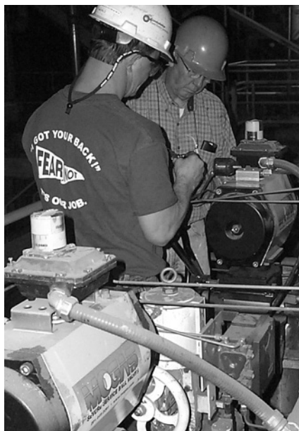
These four, 2-inch GEN-X MOGAS ball valves are handling Cold Reheat Isolation in a coal-fired plant.
